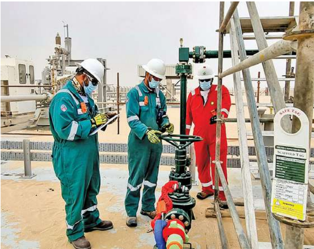
EQUIPMENT SUITABILITY: Before work began, equipment suitability and crew competency were tested by modelling different well flow situations. - Supplied picture
