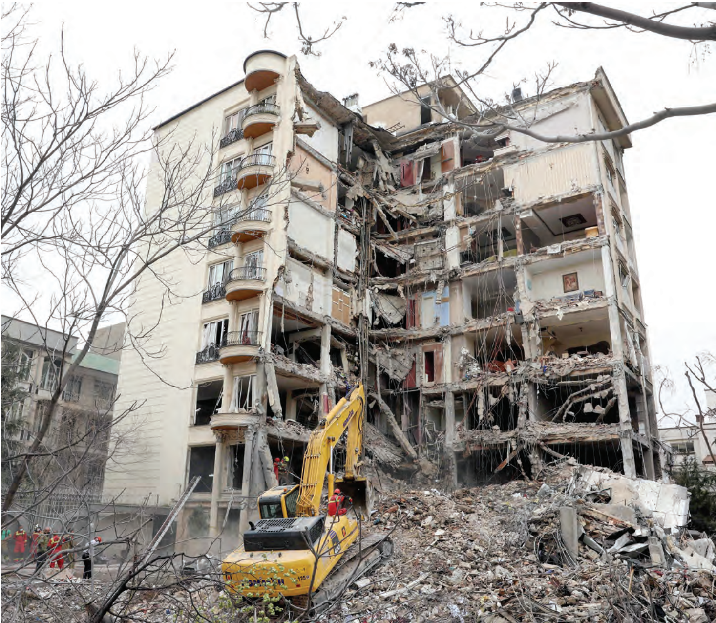
An excavator clears rubble from a destroyed residential building in northern Tehran. — AFP
