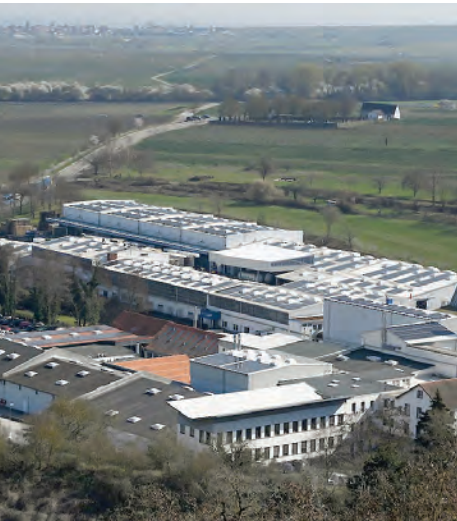
A general view of the building complex of Gechem, in Kleinkarlbach, some 25 km west of Ludwigshafen, Germany. — Reuters
