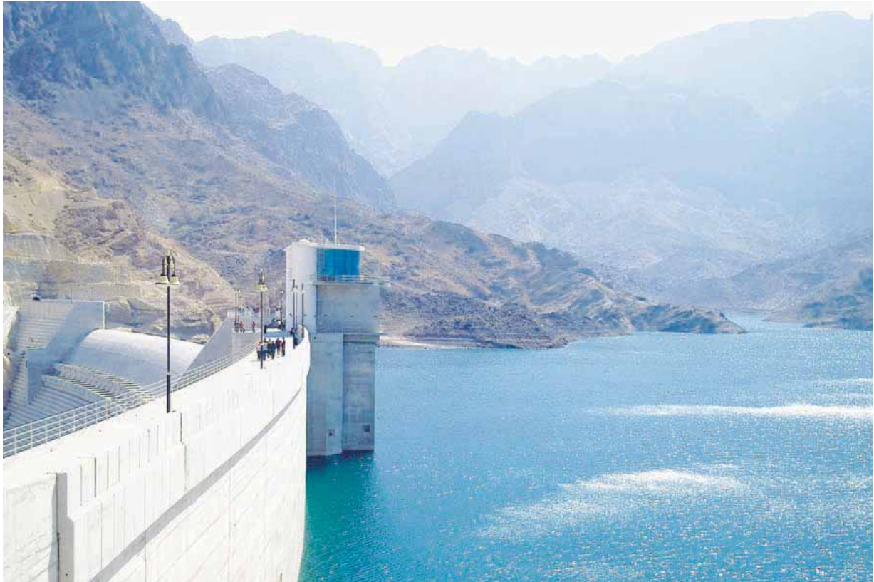
The floating solar installation at Wadi Dayqah Dam saves valuable land for agriculture and other uses, and it reduces water evaporation from the dam, which is a significant benefit.
