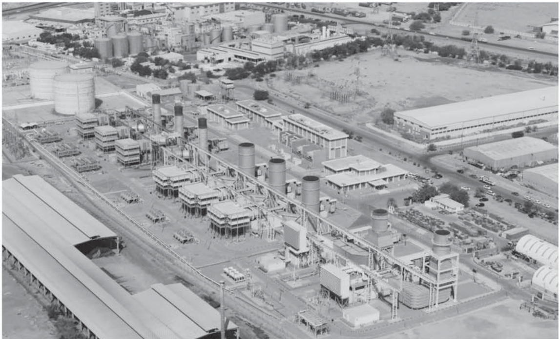
Figure 1 Al Rusail Power Plant
