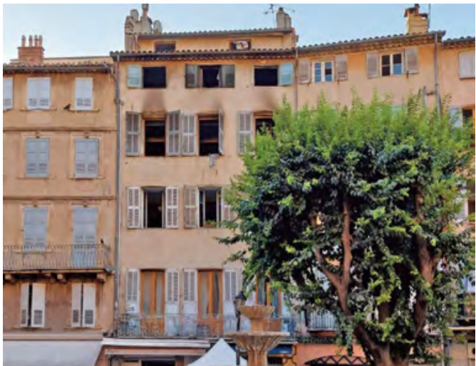
This photograph shows the burnt facade of a five-storey building in the historic centre of Grasse, on Sunday (AFP)
