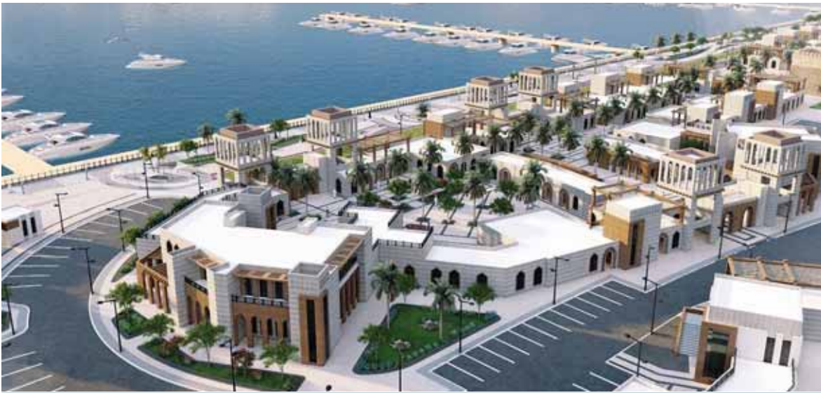
In the first phase, 95 commercial shops, 15 fish stalls, 10 restaurants and cafés, two handicraft training centres, a tourist visitor centre, a marina for fishing boats, and a hotel will be constructed
