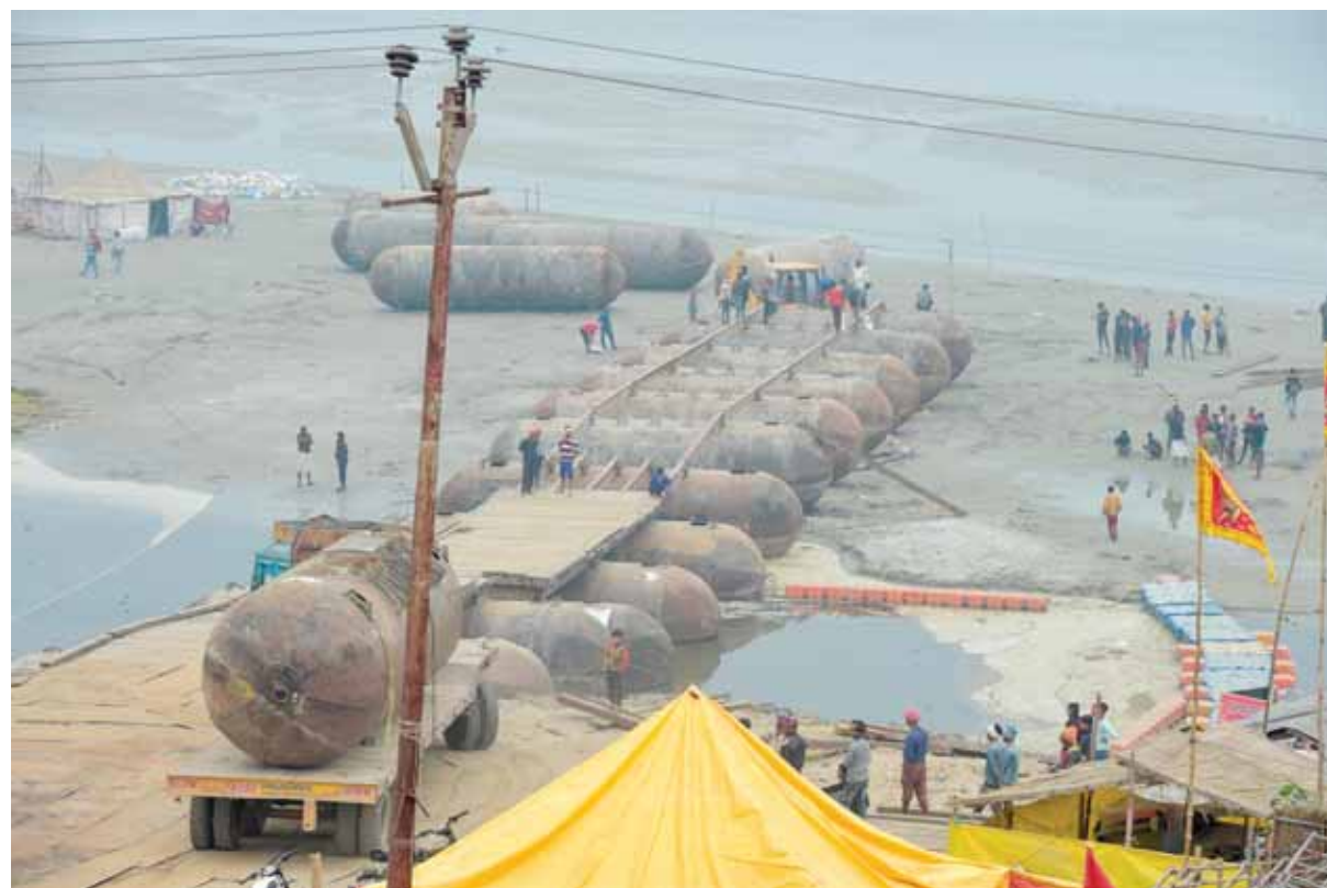
Workers build a floating bridge on the banks of the Ganges River ahead of the Magh Mela festival in Allahabad on Tuesday. — AFP
