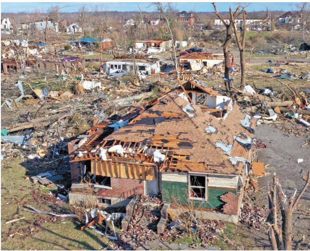
Destroyed homes after a tornado ripped through a residential area, in Mayfield, Kentucky on Saturday (AFP)
