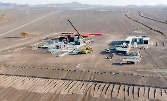
The projects are set up on an area of over 28,000 square metres.
