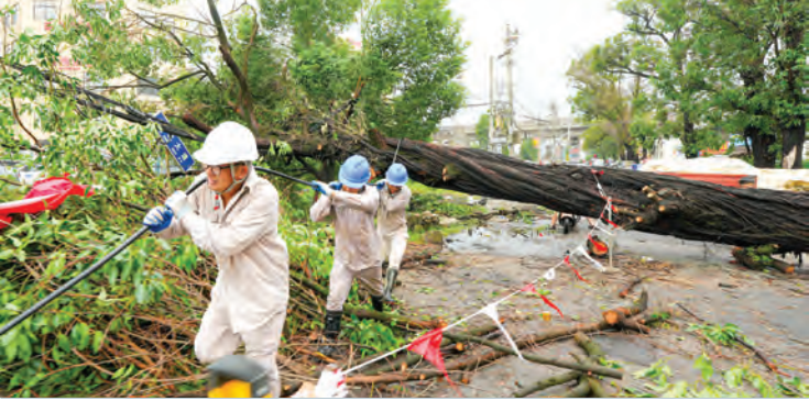
Power restoration workers clear a fallen tree and restrnging power lines in Zhejiang province, China. — Reuters
