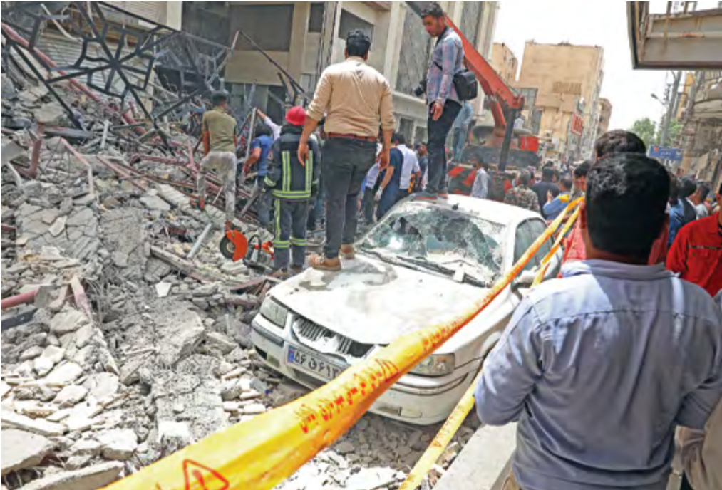
Iranians gather at the site where a building collapsed in the southwestern city of Abadan on Monday (AFP)
