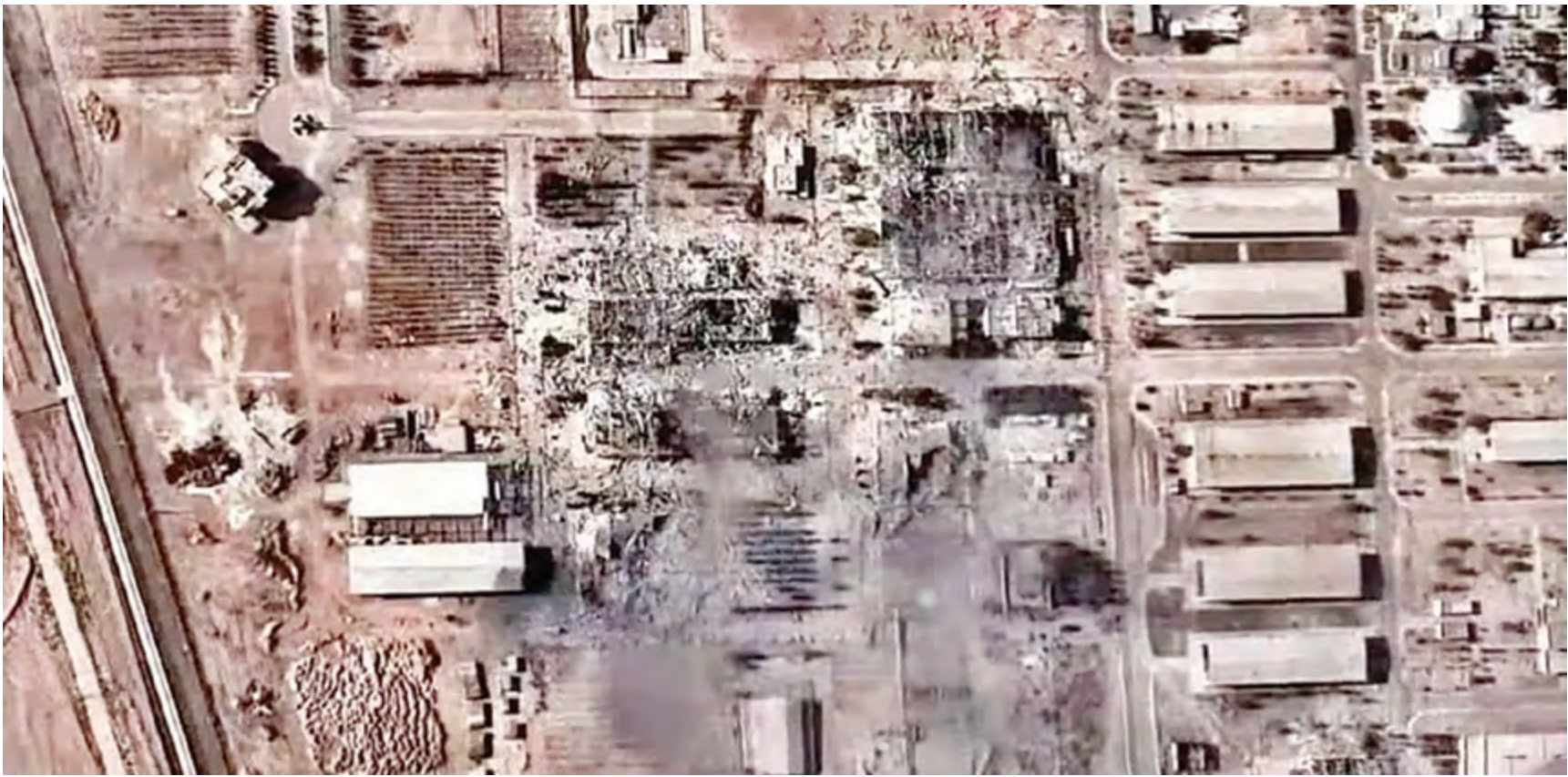
The nuclear site in Isfahan and the centrifuge production facilities that were struck on June 21
