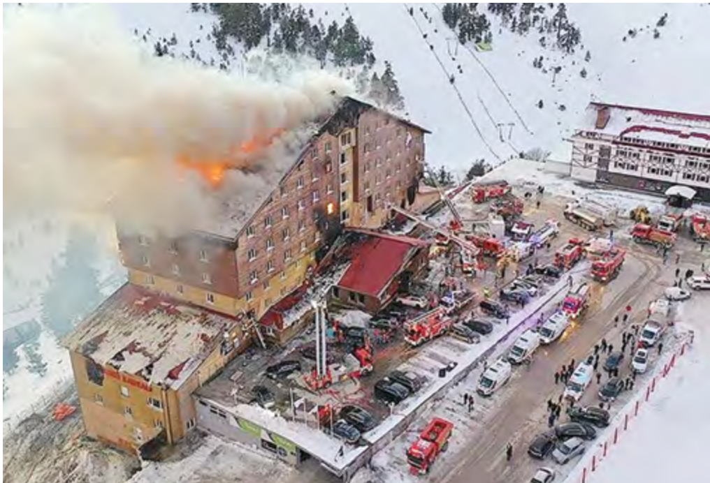
Authorities evacuated around 230 guests from the hotel as firefighting efforts continued
