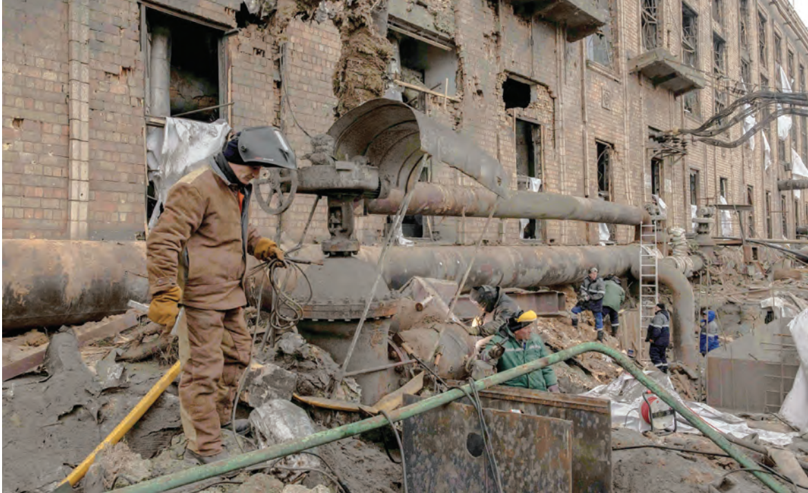
Employees repair sections of the Darnytska combined heat and power plant damaged by Russian air strikes in Kyiv on Wednesday. — AFP
