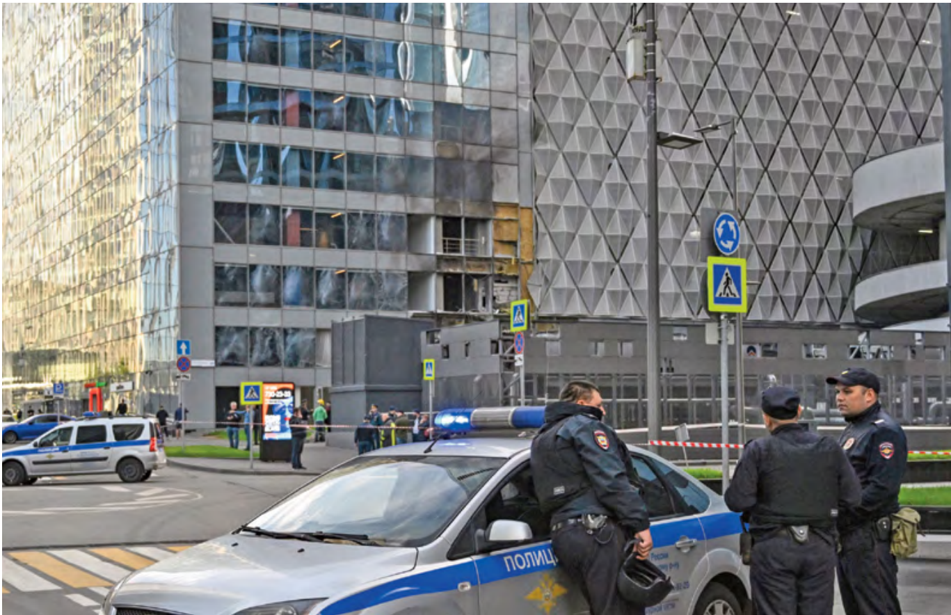
Police officers block off an area around a damaged office block of the Moskva City following a reported drone attack in Moscow on Sunday (AFP)
