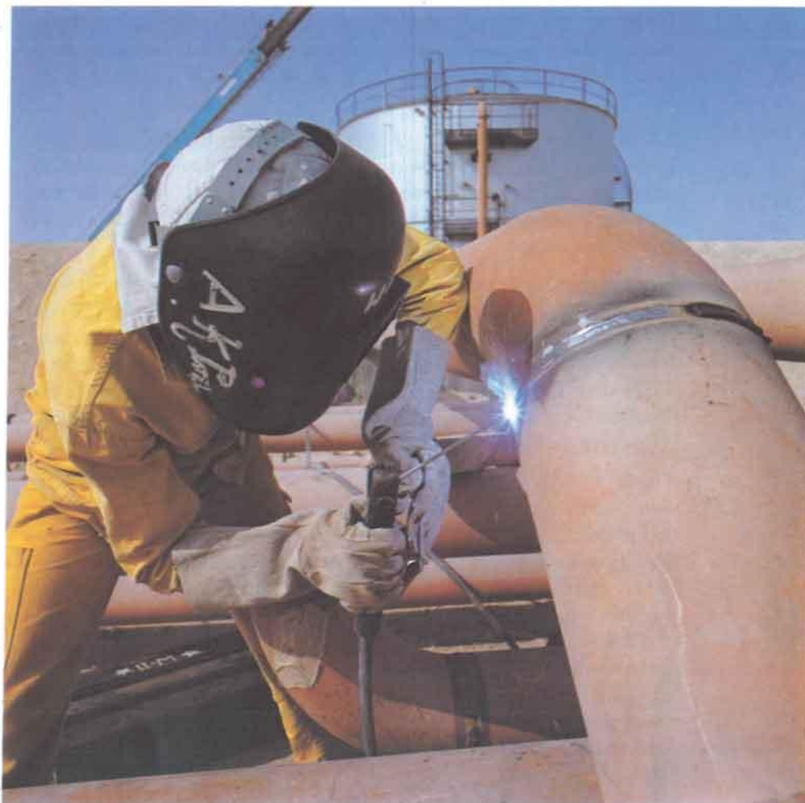
Pipeline maintenance (Photo: PDO)
