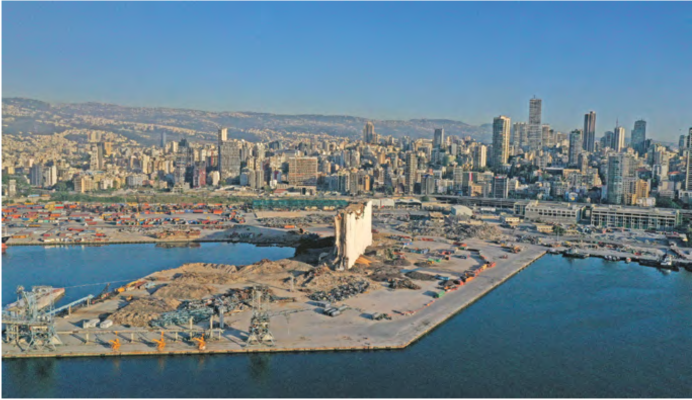
An aerial view shows Beirut port on May 27, 2021, with the grain silos in the foreground, damaged in a massive explosion on August 4 last year, which killed more than 200 people and injured scores of others (AFP)
