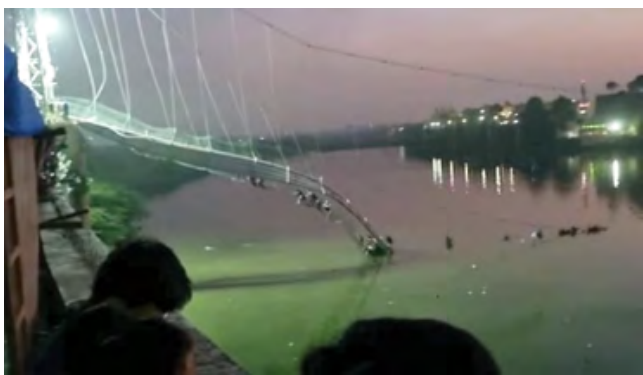
A cable bridge collapsed in the Machchhu river in Morbi district
