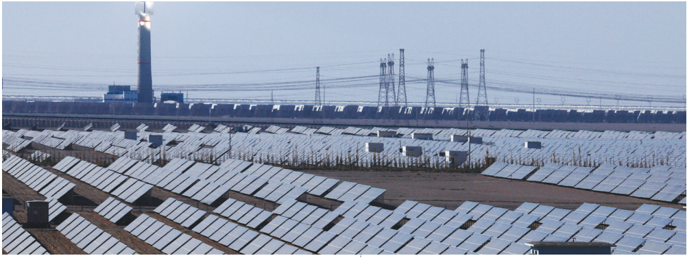
A general view of solar panels at the Dunhuang Photovoltaic Industrial Park in Gansu province, China. — Reuters
