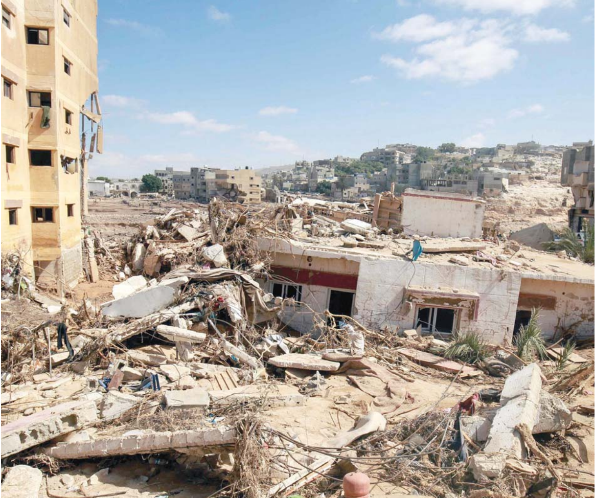
The rubble of buildings that collapsed during floods are piled up after the Mediterranean storm “Daniel” hit Libya’s eastern city of Derna. – AFP
