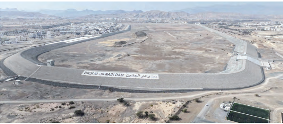
It took three years to implement Wadi Al Jifnain Dam project.
