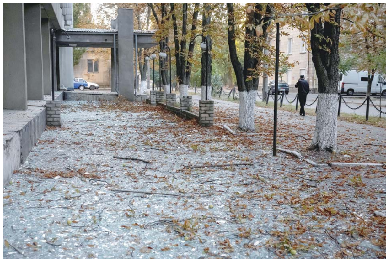
Broken windows are seen near a building damaged during a Russian drone strike, amid Russia's attack on Ukraine, in Kyiv. — Reuters
