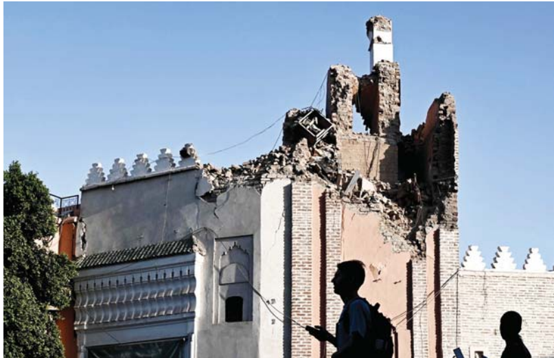
People walk past a damaged building in the old quarters of Marrakesh. — AFP
