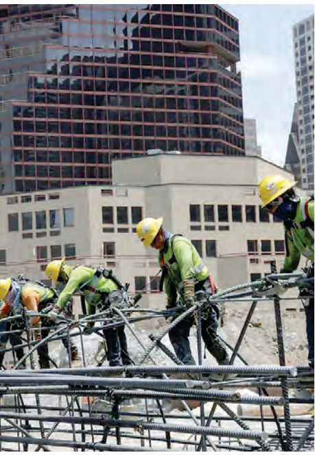
Construction workers are seen at a residential housing development in San Diego, California. — Reuters
