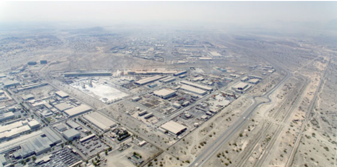
EXPANSION: Madayn is completing the infrastructure works for the expansion of phase 7 in Sohar Industrial City at a total cost surpassing OMR13 million. - Supplied picture
