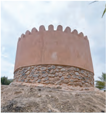
The restoration works encompassed structural reinforcement of the tower.
