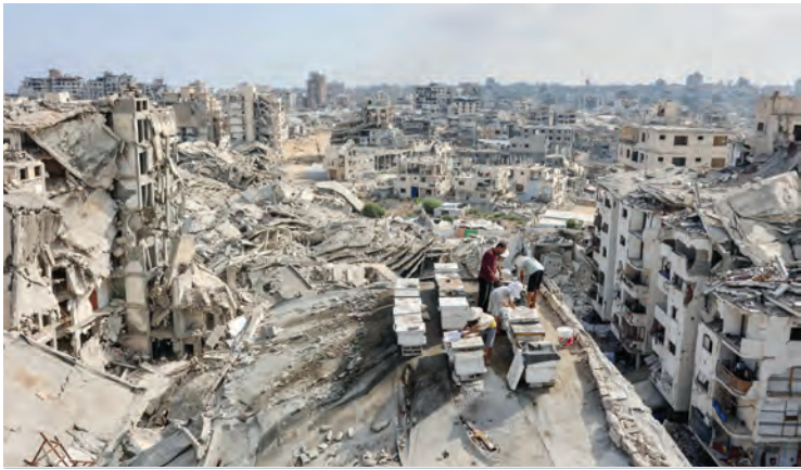
Ibrahim al Dabba, head of the Beekeepers Cooperative in the Gaza Strip, tends to beehives with his sons on the roof of a destroyed building in Gaza City’s Tel Al Hawa neighbourhood, where the displaced family has taken refuge, on Wednesday. — AFP
