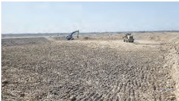
The completion rate of construction work in the first phase of the whiteleg shrimp farming project in Shinas has reached 80 per cent. — ONA
