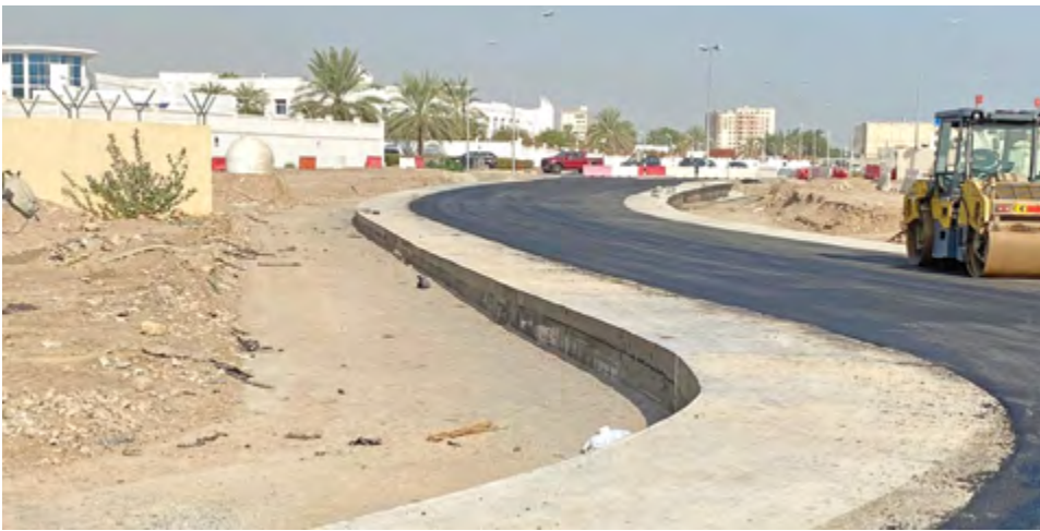
Muscat Municipality has stated that it completed 85 per cent of the road project linking several streets in the southern Ghubra area of Bausher. The project includes laying a road network in the area with oil and gas lines underneath, transferring existing public services, and constructing a water canal (Supplied photo)
