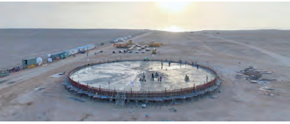
Construction work underway at ACME's green hydrogen and ammonia project in Duqm SEZ.
