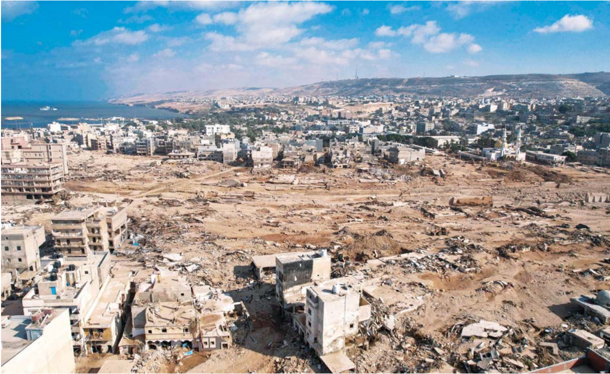
An aerial picture shows a view of the damage in the aftermath of a devastating flood in eastern Libya’s city of Derna. – AFP
