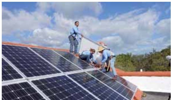
Workers install solar panels on a rooftop at a home in Palmetto Bay, Florida. — AFP
