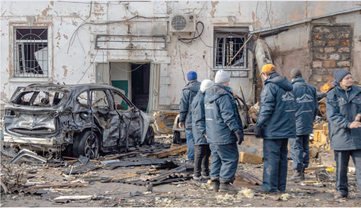
Communal workers stand next to burnt cars in the courtyard of a building damaged as a result of a drone attack in Odesa. — AFP
