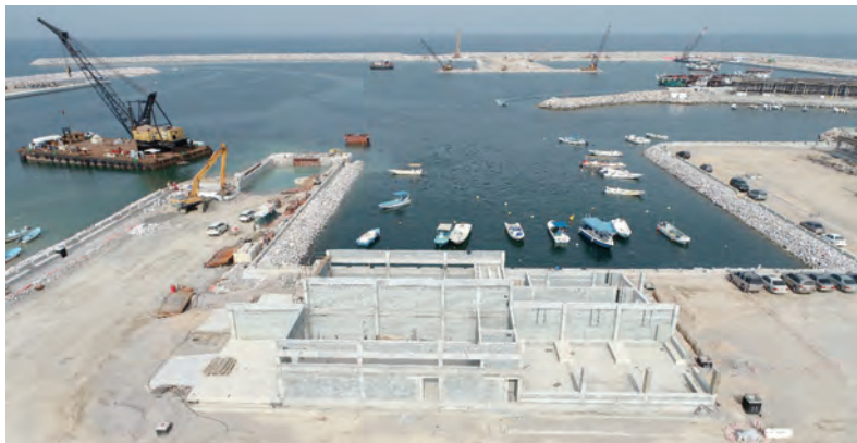
The construction work on the Dibba Port is well in progress with the completion rate at 75 per cent
