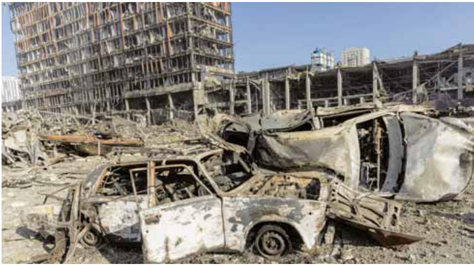
A view of the site of a bombing at a shopping centre as Russia's attack on Ukraine continues in Kyiv.
