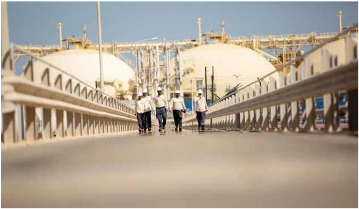
Methanation will help with Oman LNG's decarbonisation goals, as well as the production of greener LNG fuels.
