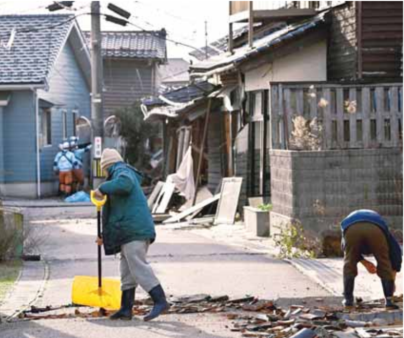
Residents clean up debris in Wajima, Ishikawa prefecture on Tuesday, a day after a major 7.5 magnitude earthquake struck the Noto region in Ishikawa prefecture in the afternoon. – AFP
