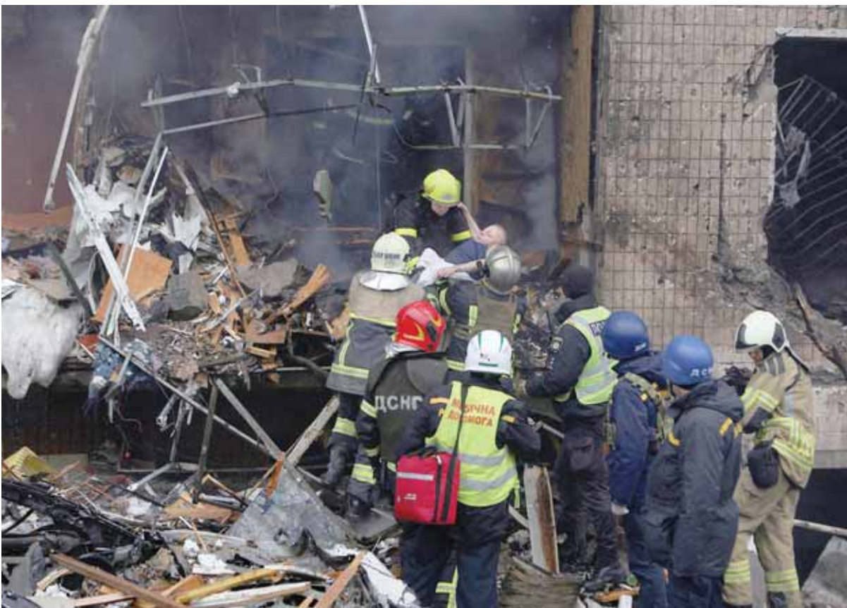
Rescuers evacuate a local resident from a residential building heavily damaged during a Russian missile attack, in Kyiv, Ukraine. — Reuters
