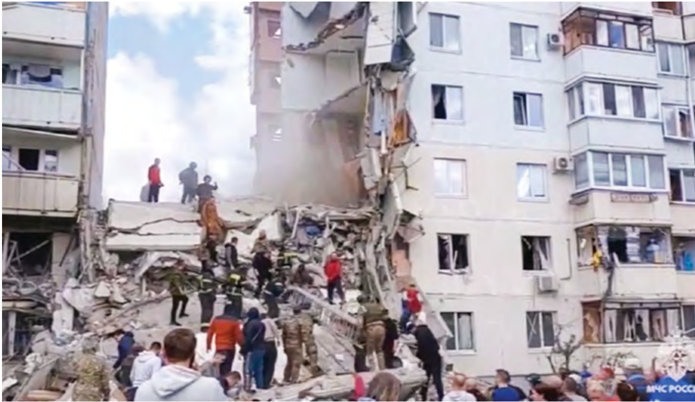
Rescuers working at the scene of a collapsed residential building in Belgorod, Russia on Sunday (Xinhua)
