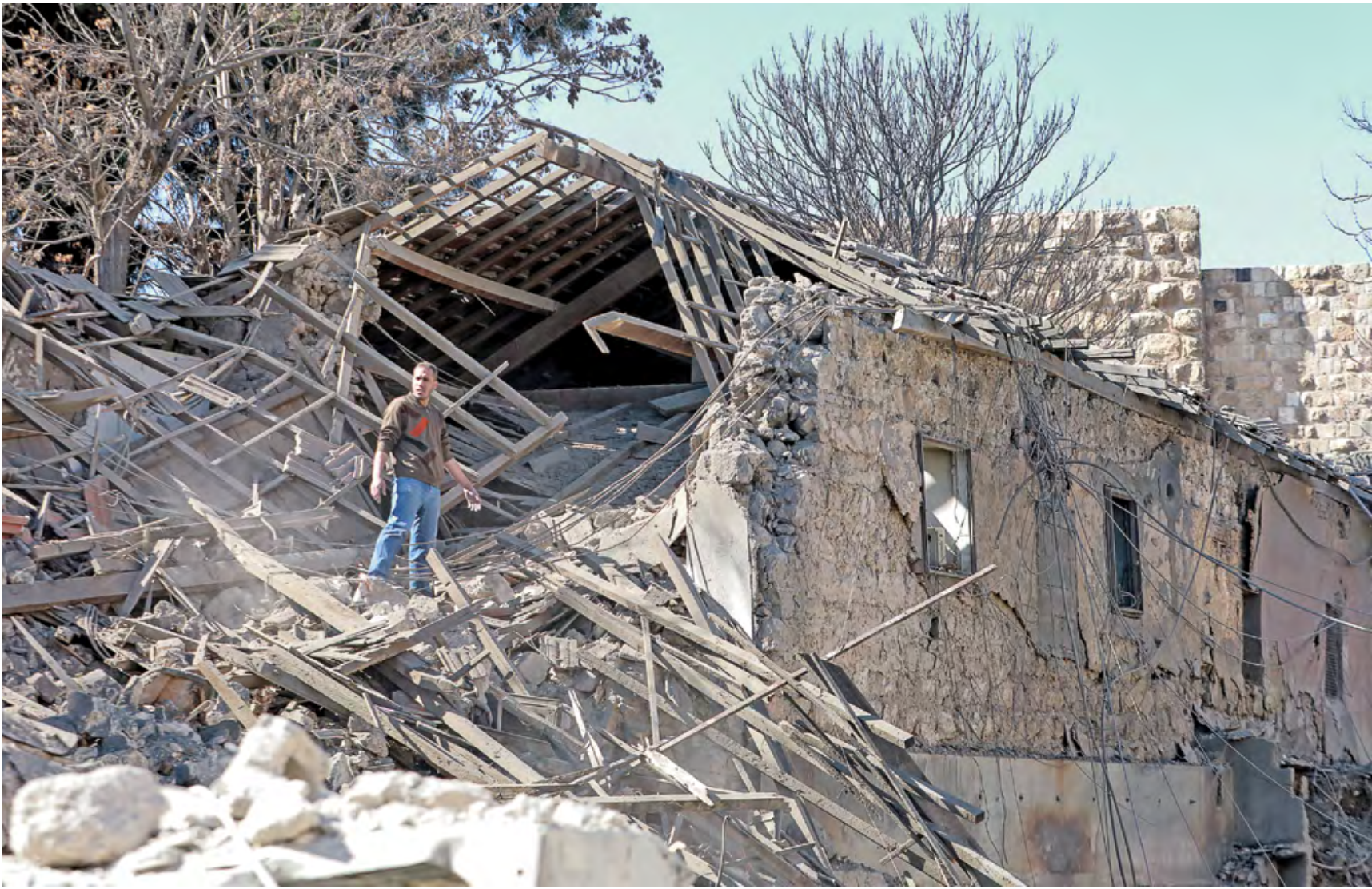
A man inspects damage in the aftermath of an Israeli air strike that hit the medieval Citadel of Damascus on Sunday (AFP)
