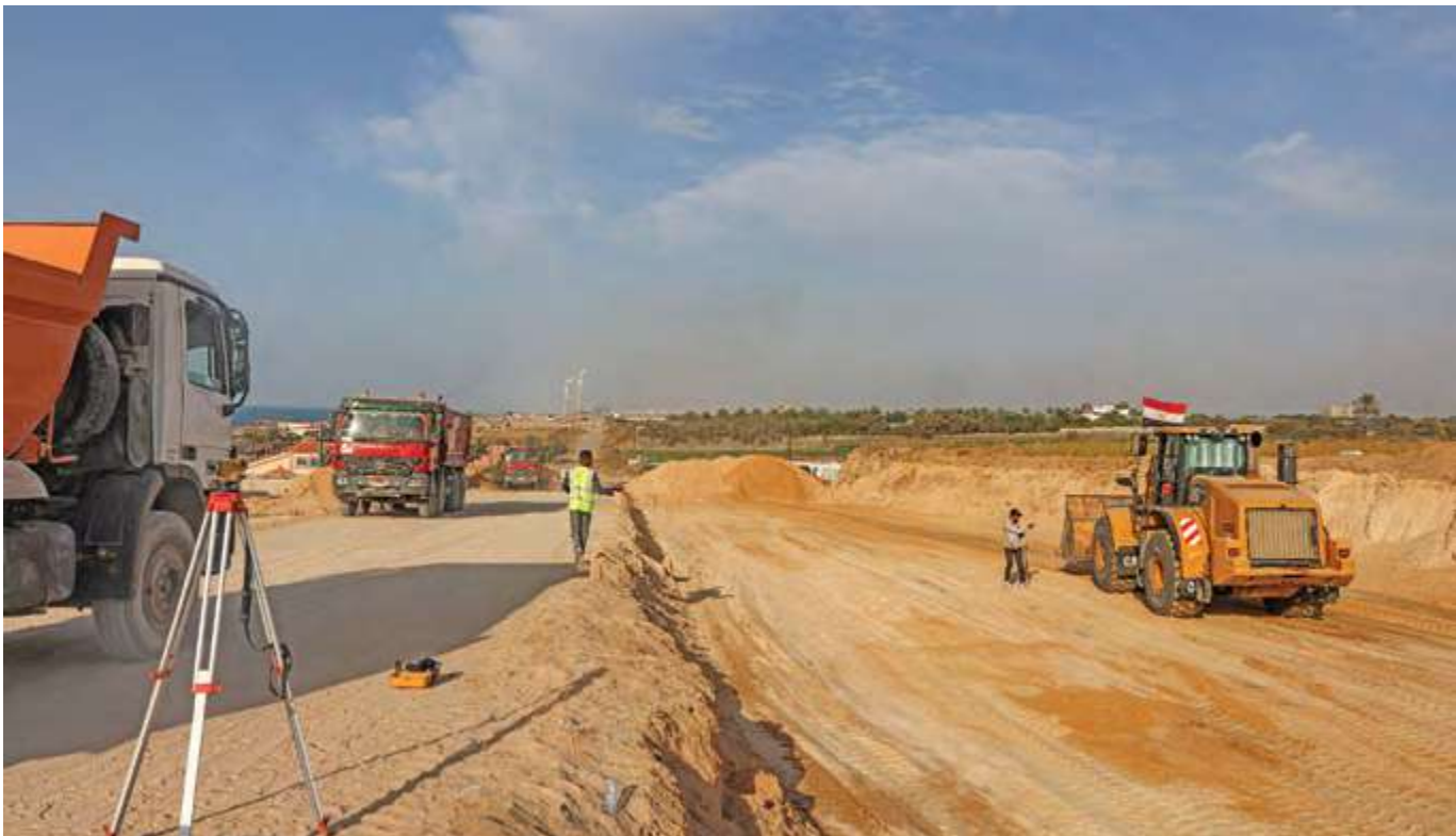
An excavator clears land at a road section undergoing expansion north of Gaza City on October 30 (AFP)
