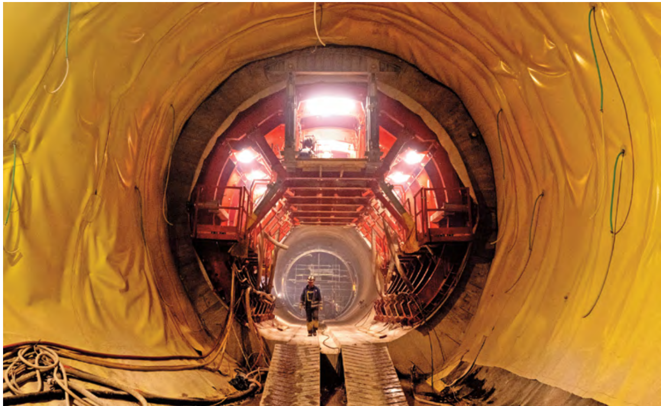
A construction site under the earth near Kaprun, Austria
