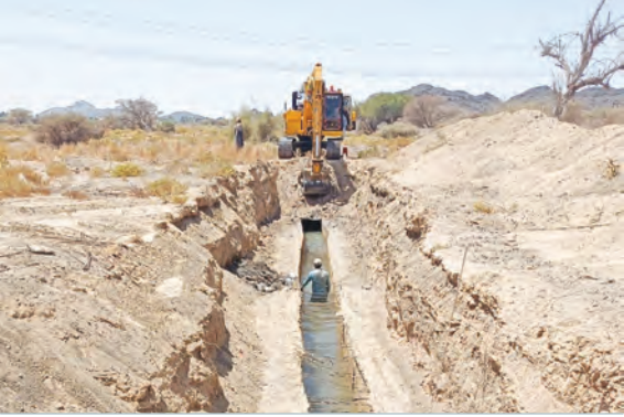
The aflaj restoration project is worth over RO 2 million
