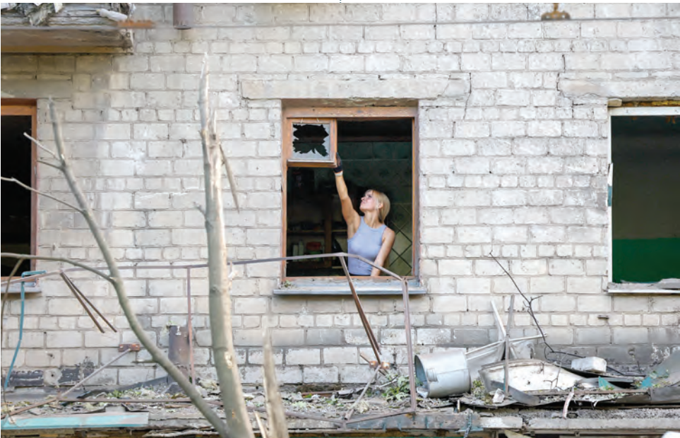
A woman removes a broken glass in a damaged apartment building. — Reuters
