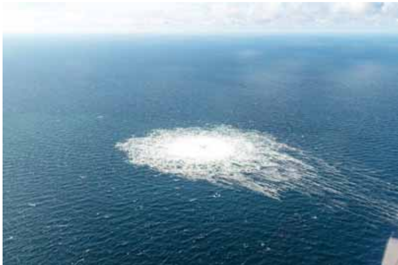
Gas leak from Nord Stream 2 pipeline as seen from a Danish F-16 interceptor jet over Bornholm island, Denmark. — Reuters file photo
