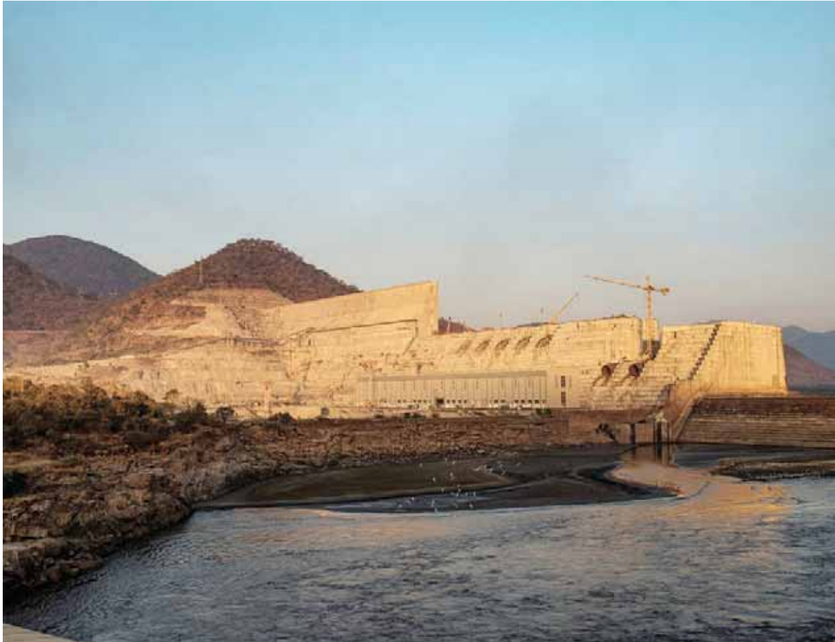
This photo taken on December 26, 2019, shows a general view of the Grand Ethiopian Renaissance Dam (GERD) under construction, near Guba in Ethiopia. — AFP
