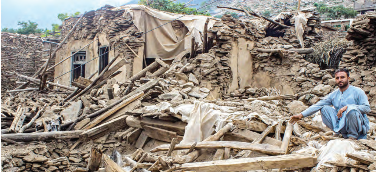
A man sits amid the remains of a damaged house in the aftermath of an earthquake at the Darai Nur district of Nangarhar province on Wednesday. — AFP
