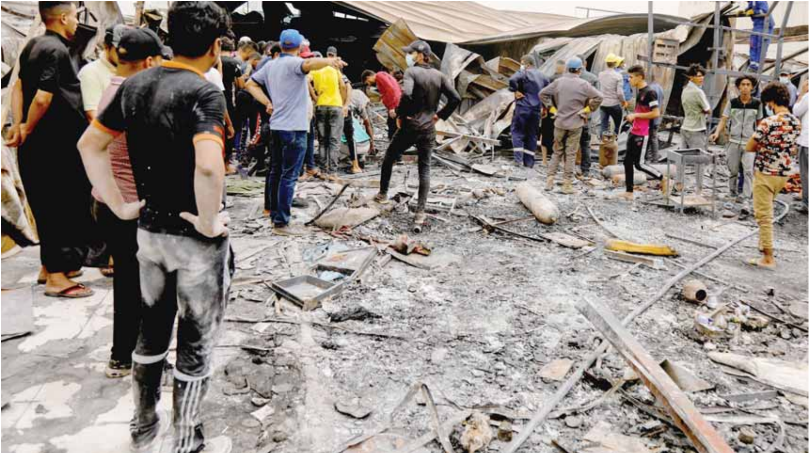
People gather as they inspect the damage at Al Hussain coronavirus hospital. — Reuters
