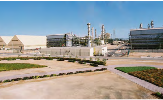
OMIFCO owns and operates a major ammonia and urea fertiliser production plant at Sur.
