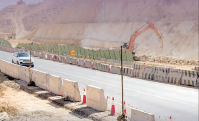
The project includes converting existing roundabouts into bridges and tunnels.
