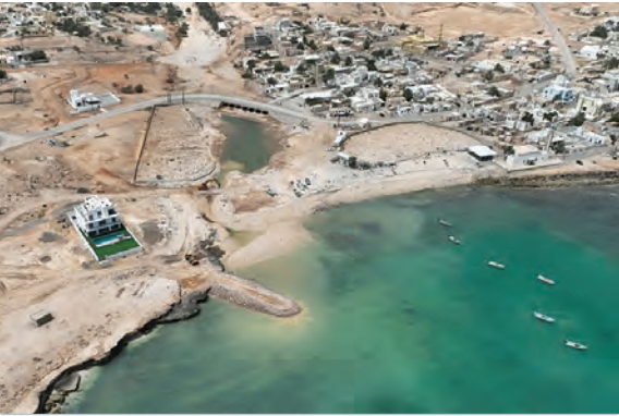
The project includes construction of breakwaters to protect boats.
