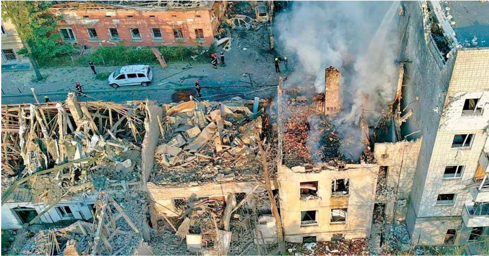
A drone view shows residential buildings heavily damaged during a Russian drone and missile strike amid Russia's attack on Ukraine in Lviv, Ukraine. — Reuters
