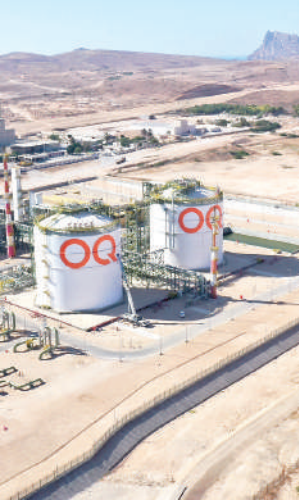
OQBI boasts a combined nameplate production capacity of 1,816 ktpa across its methanol, ammonia and LPG production plants in the Salalah Free Zone.
