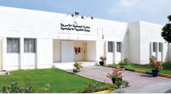
The protection shelter is an integrated institution concerned with providing care
