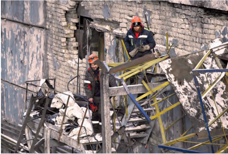
Workers clear debris at a heavily damaged thermal power plant in an undisclosed location in Ukraine. — AFP
