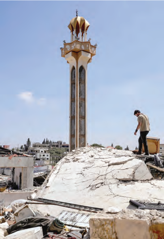
A man inspects the damage at a mosque in Jibchit, Nabatieh district, Lebanon. — Reuters
