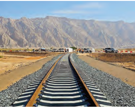
Hafeet Rail Project 40% complete.
